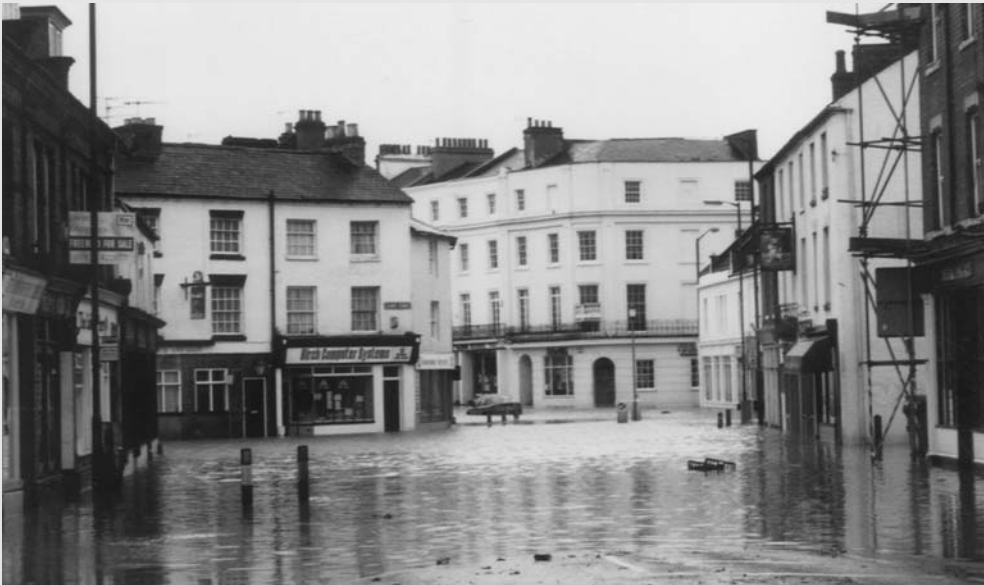
▲ 1.5 Flooding in central Leamington
