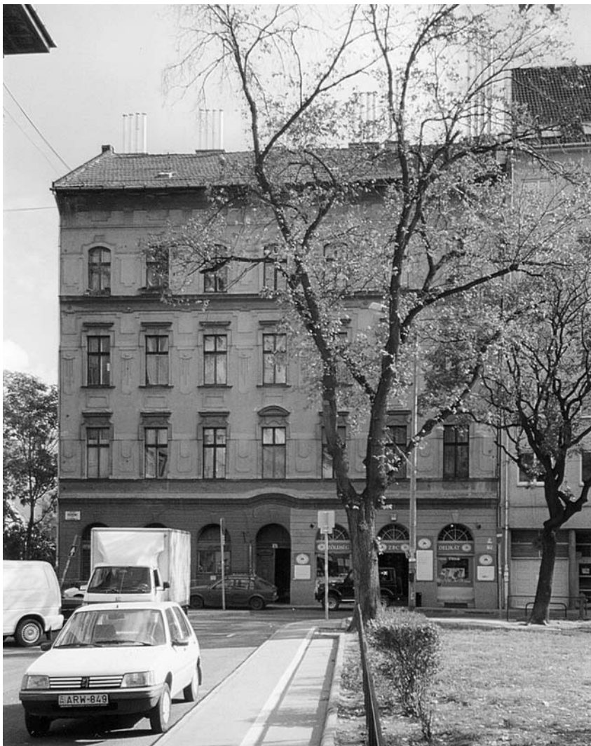
▲ M1 Renovated tenement
