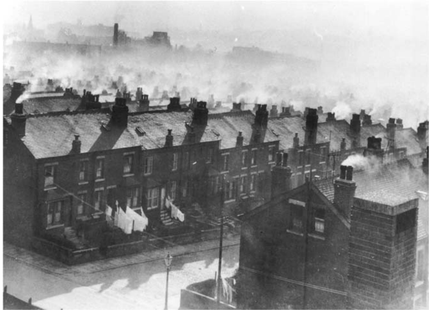
▲ 0.2 Back-to-back housing in Leeds
