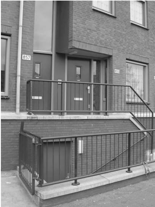
▲ K7 Entrances to upper and lower maisonette and access to basement storage
