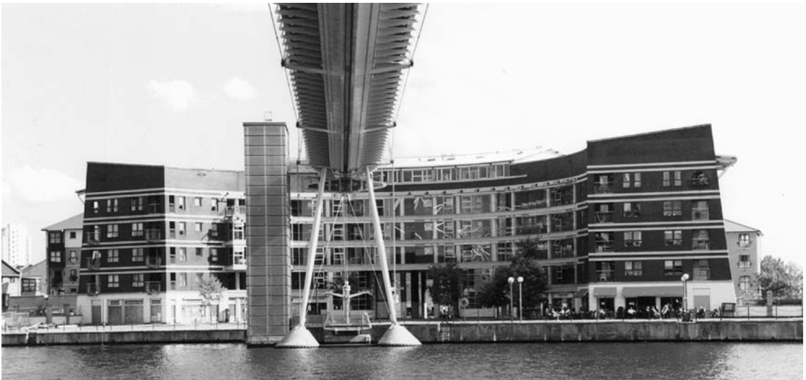
▲ C5 The Crescent building and footbridge over the dock
