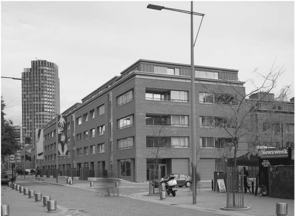
▲ A2 The ‘hard’ public face of the scheme clad in brickwork
