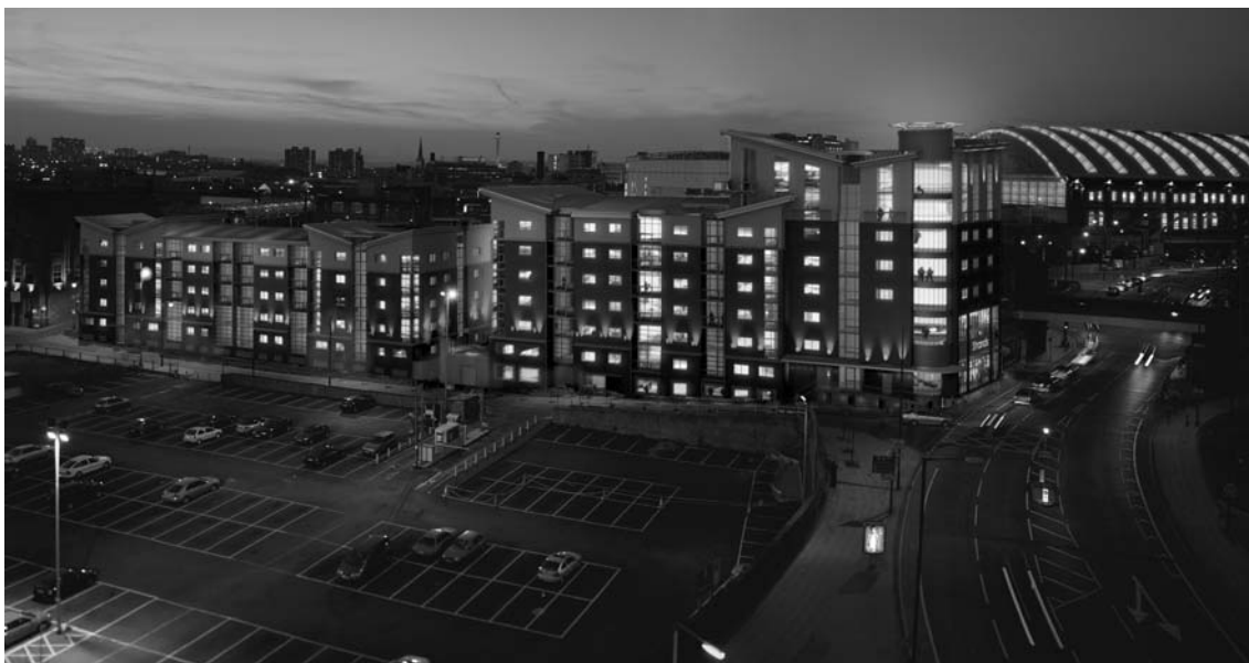
▲ B1 Overall view of the development
