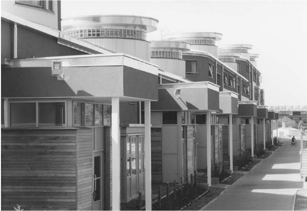
▲ G5 'Passive-stack' vent turrets to staircases
