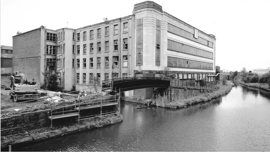
▲ 6.11 The factory before conversion
