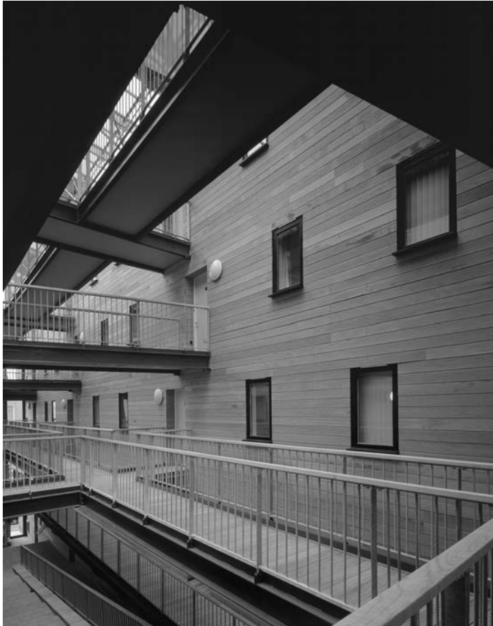
▲ F7 Bridges to the individual flats
