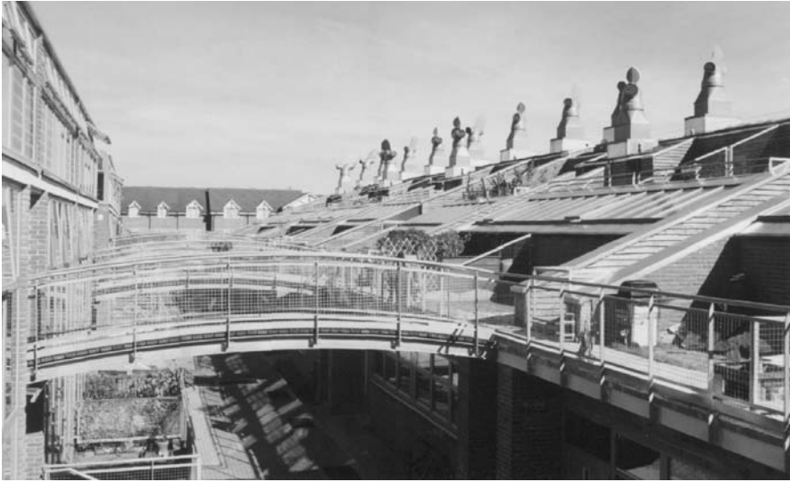
▲ H6 Gardens on top of workspaces reached by bridges over access road
