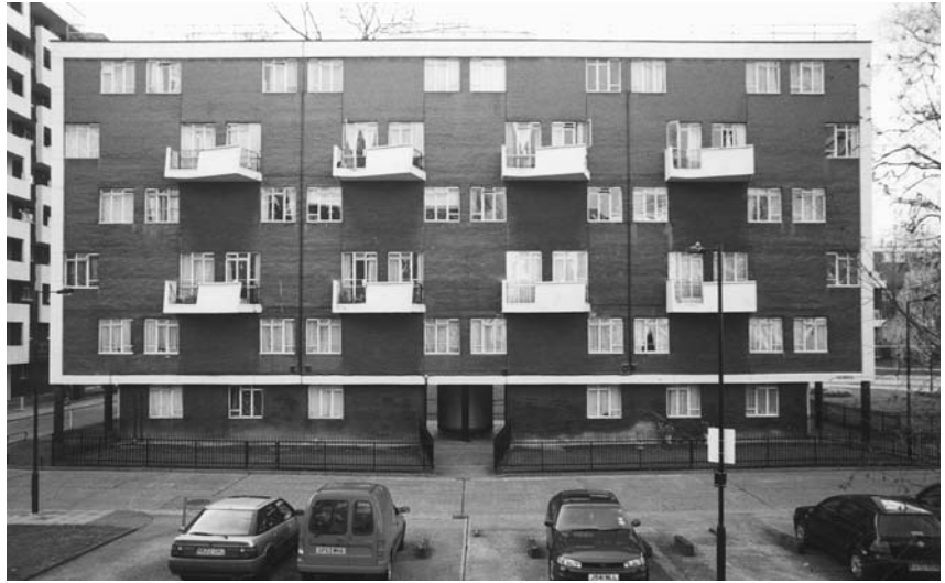
▲ 7.2 Hallfield estate, London W2 – Façadeism. Balconies are used chiefly to make a façade pattern so only some of the flats in the block have the benefit of private outdoor space
