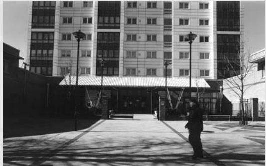
▲ 6.6 The new secured main entrance
