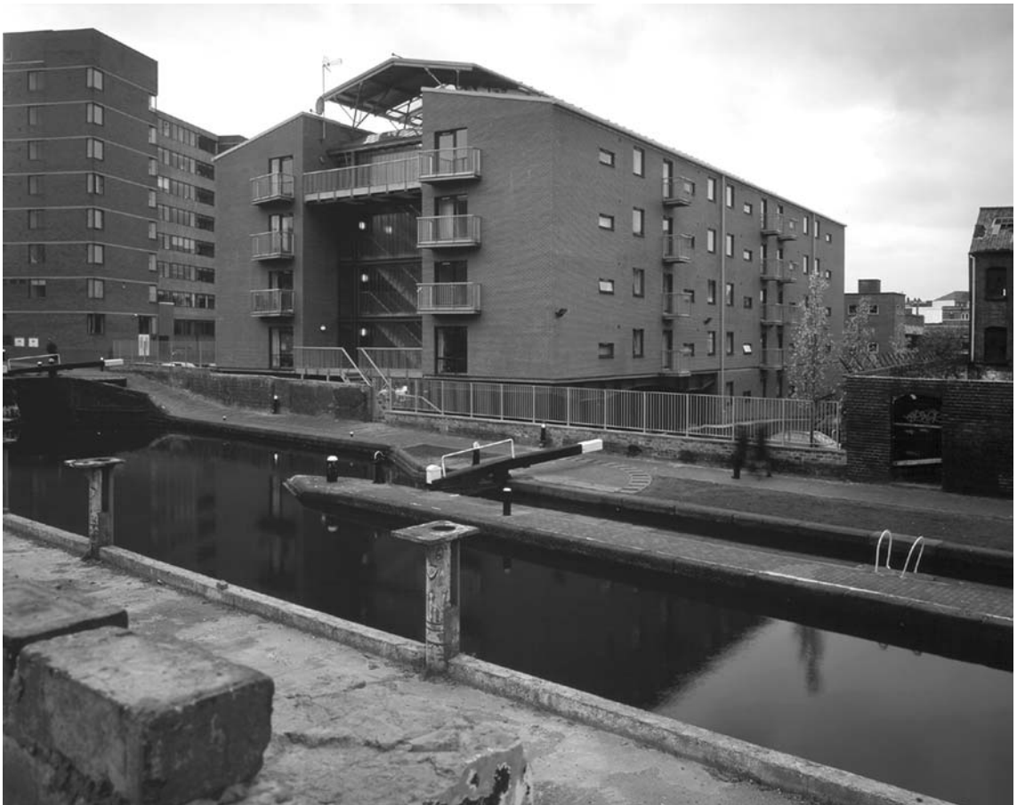
▲ F1 The canal-side frontage of the building
