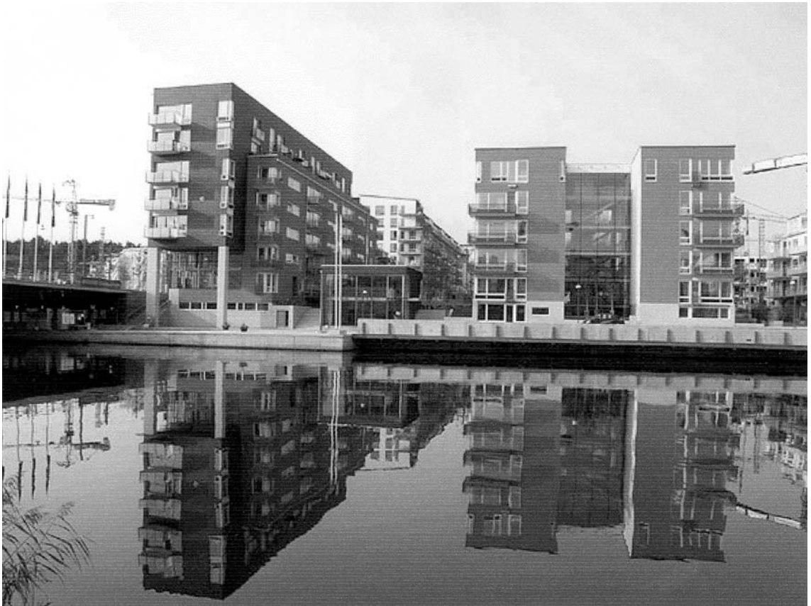
▲ L1 Harbour-front blocks in phase 1
