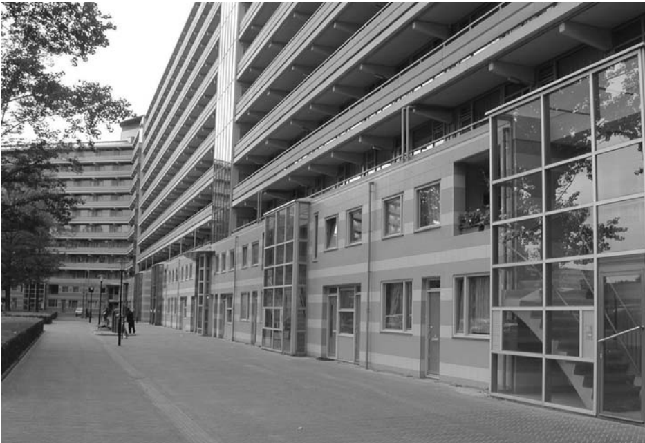
▲ K2 New maisonnettes and entrances built into lower levels of multi-storey block
