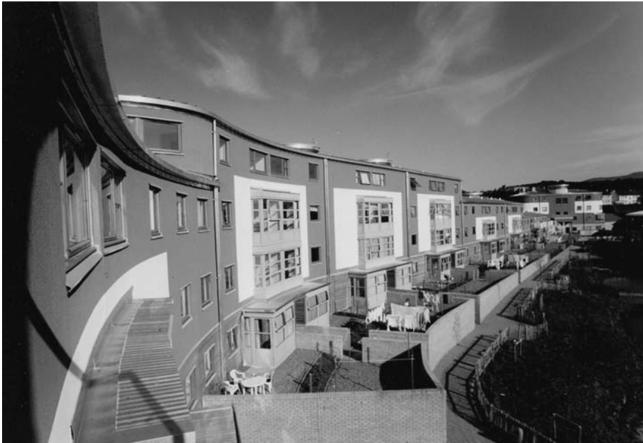
▲ G6 The central space, ponds on the right
