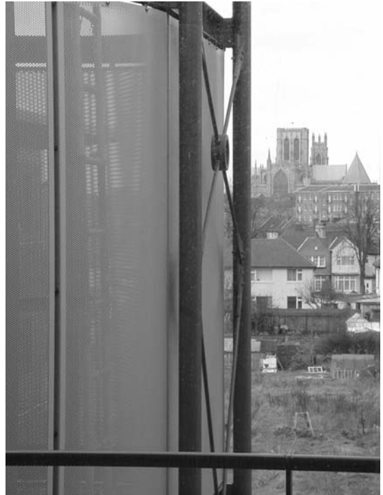
▲ 14 York Minster viewed alongside lift/stair enclosure
